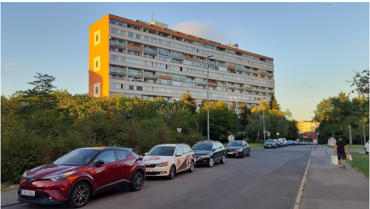
Figure 10.4: Maisonette flats at Krč housing estate.
