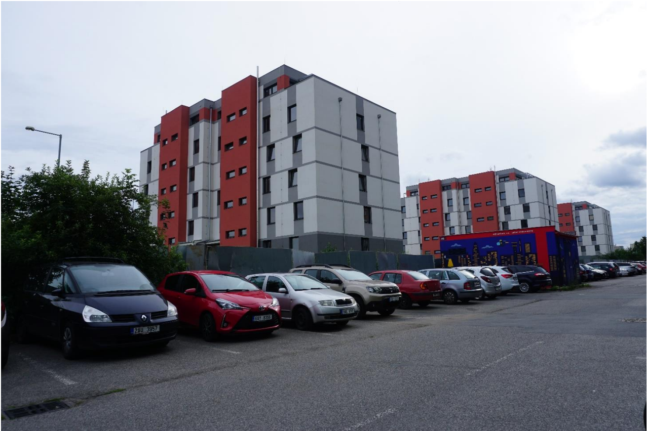
Figure 15.4: Černý Most II—New construction on Bryksova Street.
