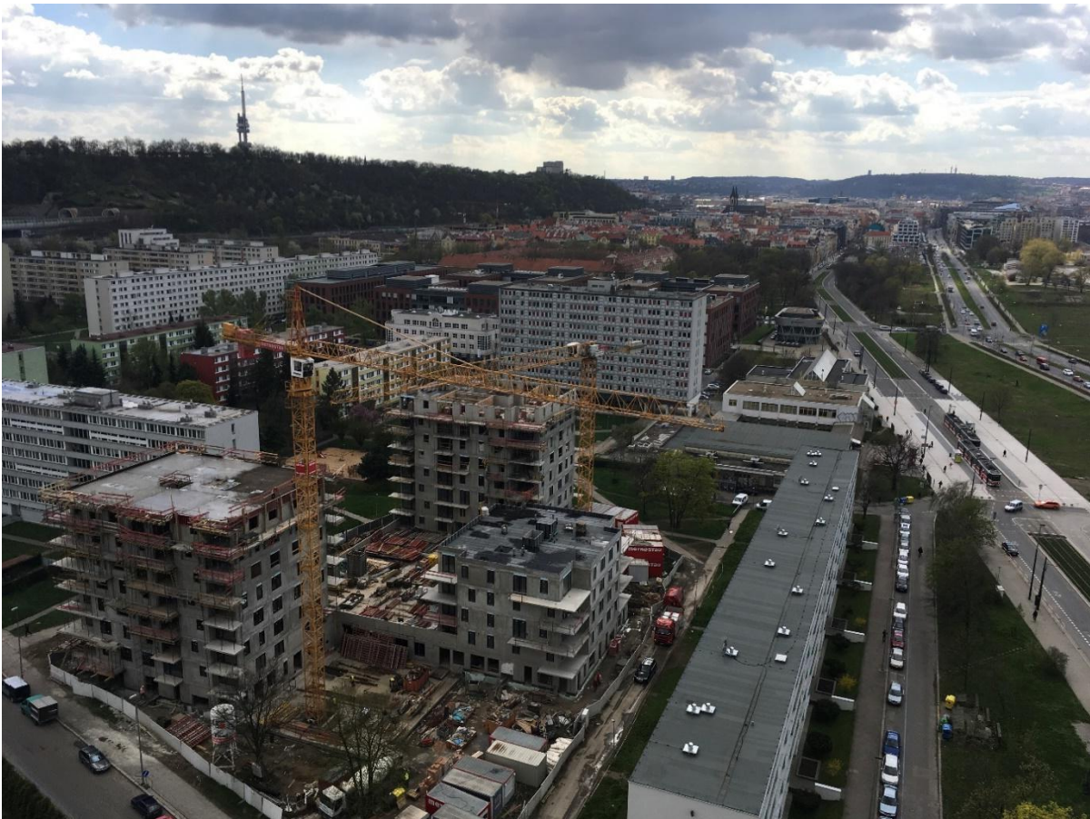
Figure 2.4: In the core of the Invalidovna housing estate, a new residential project is being built on the site of the former kindergarten. Behind the hotel building is the Futurama office complex. On the far right is Pobřežní Street, which separates the new development on Rohan Island from old Karlín.
