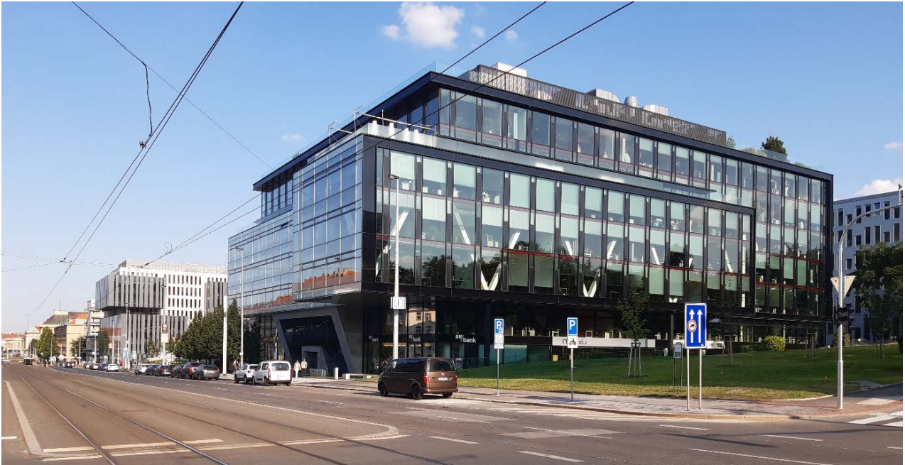
Figure 6.2: Administrative complex PPF Gate on Evropská street.
