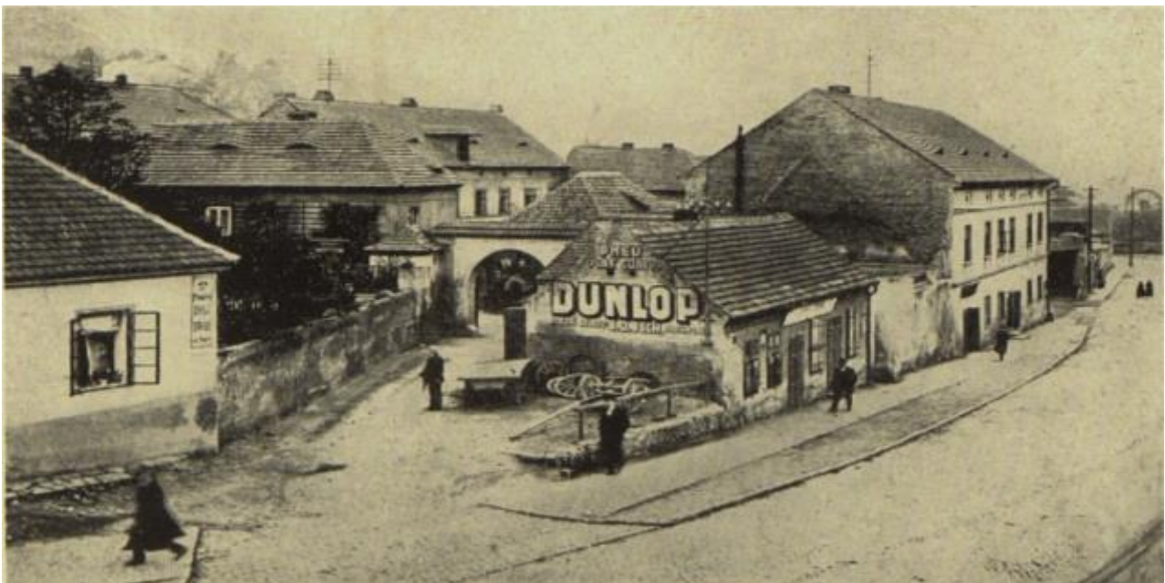
Figure 13.2: Zlíchov at the beginning of the twentieth century.
